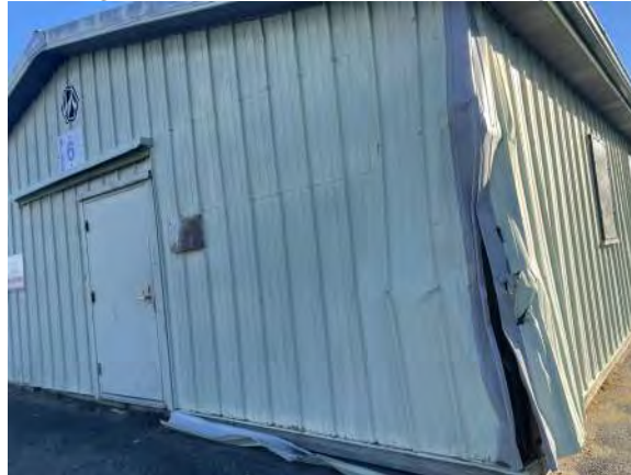
Figure 3.2.7 Exterior of the Morton Building 12
