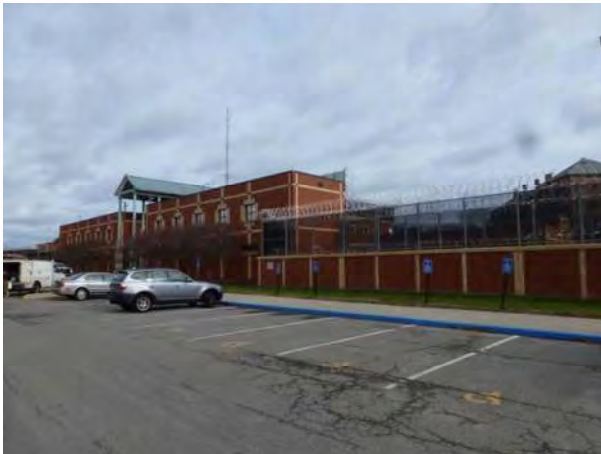
Betty Cole Smith Building, view northeast
