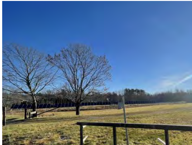
Figure 3.1B Solar Panel Field from a distance 12
