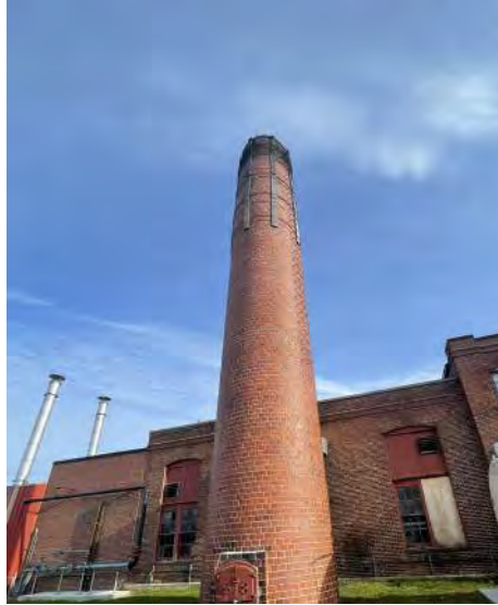
Figure 1.3.10.2 Power Plant - Top of chimney braced by wooden slats and metal wiring 3
