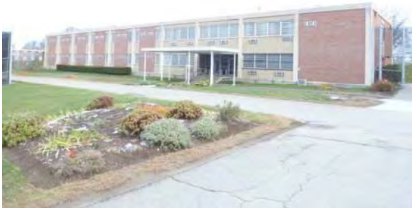
Health Services Building, view northeast
