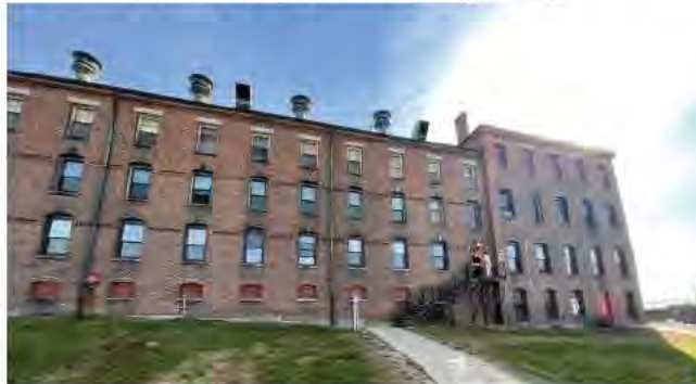
Figure 1.3.7 Old Administration Building 3
