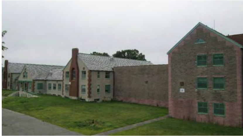
Figure 3.2.4 Administration Building (left) and the Main Building addition (right) 11
