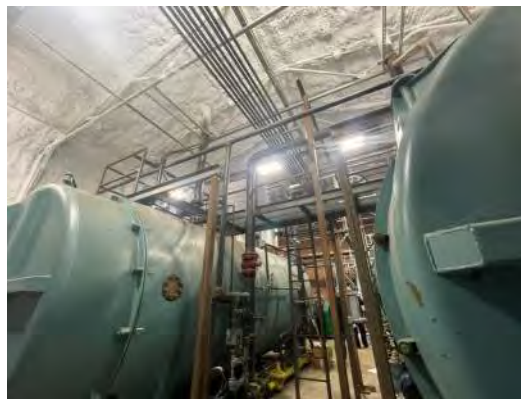
Figure 1.3.10.3 Power Plant - New Boiler Room addition 3
