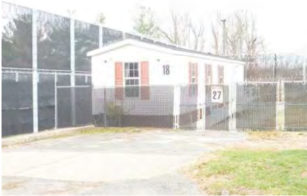
Vinyl Clad Building, view north
