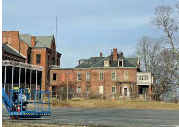
Figure 1.3.6 Old Superintendent's House fenced off 3
