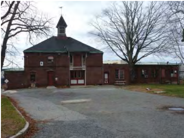
Garage/Carpenter's Shed, view west
