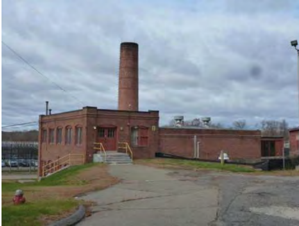
Power Plant, view west
