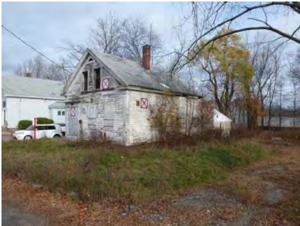
364 Irving Street (FRM.304), view northeast
