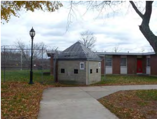
Pump House, view east
