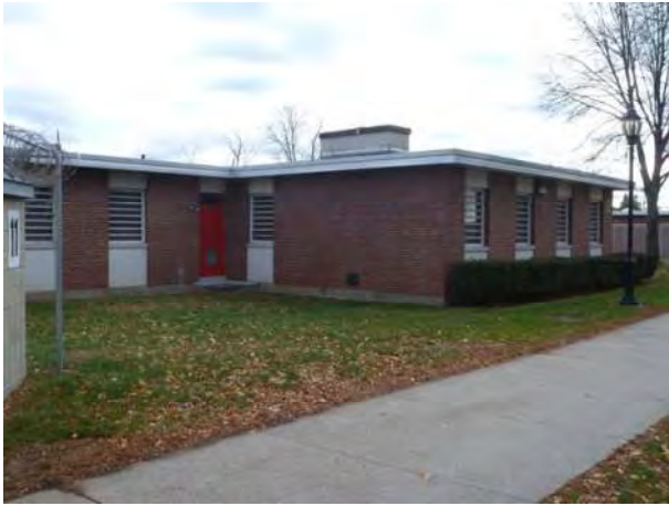
Townline, view east
