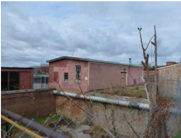
Tool Crib, view northwest
