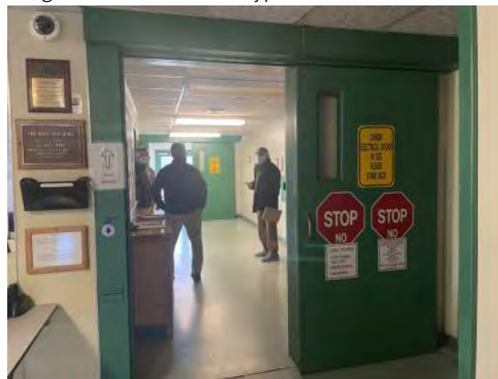
Figure 3.3.1.2 Internal sallyport in the Gate House 12
