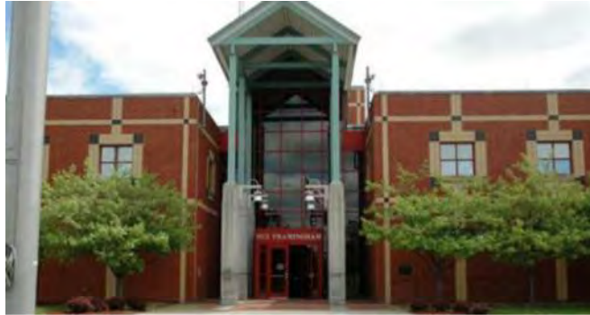
Figure 1.3.1 Front entrance to the Betty Cole Smith Building 7
