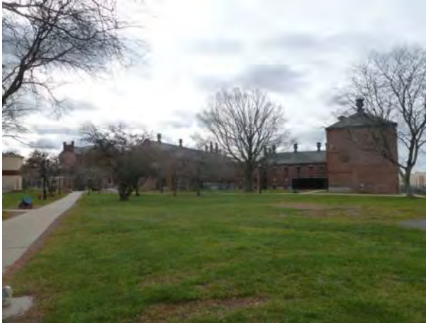
Old Administration Building, view southwest
